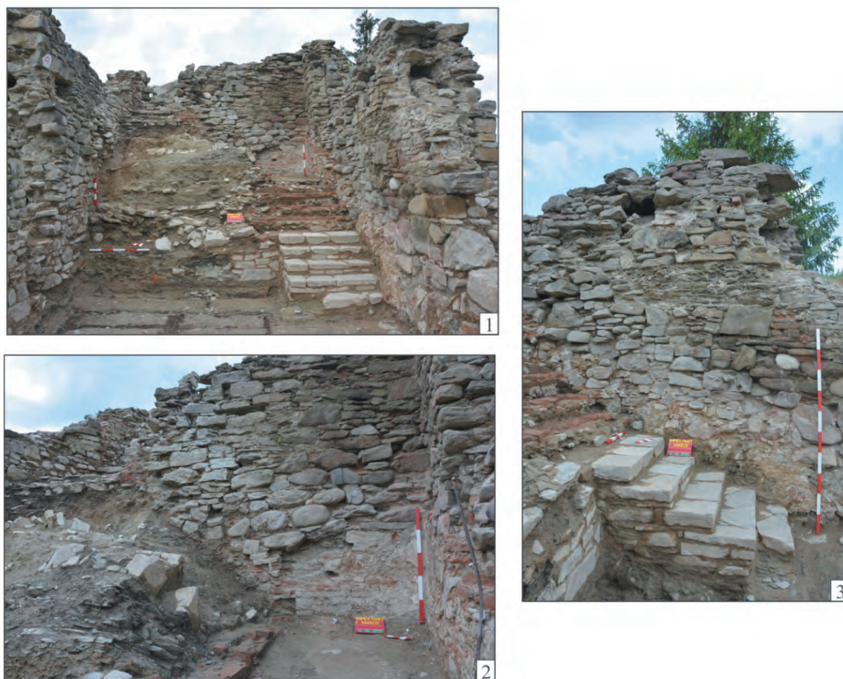
Fig. 7. Ghimeș-Făget. The former customs point “Cetatea Rákóczi” (area B). 1, 3. Details of the stone and brick steps; 2. The dividing wall of the fortification with the imprint of the wooden steps. View from the east.
