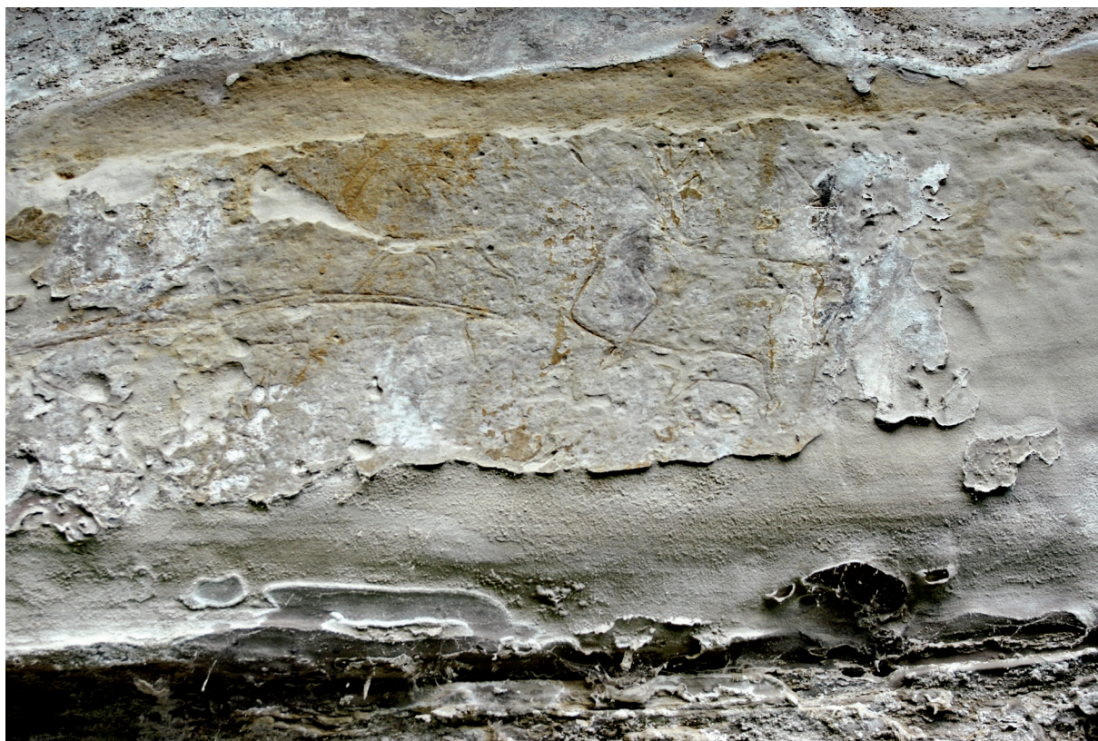
Fig. 9. Area 3 – general view
